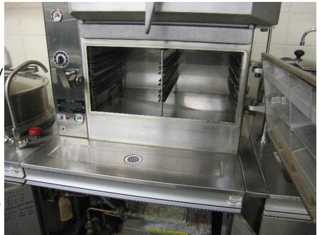
In most cases, it was hot water contact that caused the injuries. Excessive hot water built up on the interior of the steamers and when the door was opened, it spilled onto the adjacent table. The table drain was unable to handle the volume of water coming out of the steamer, causing it to overflow. The employees, in an attempt to minimize spillage, burned their hands, legs and feet in the process.
